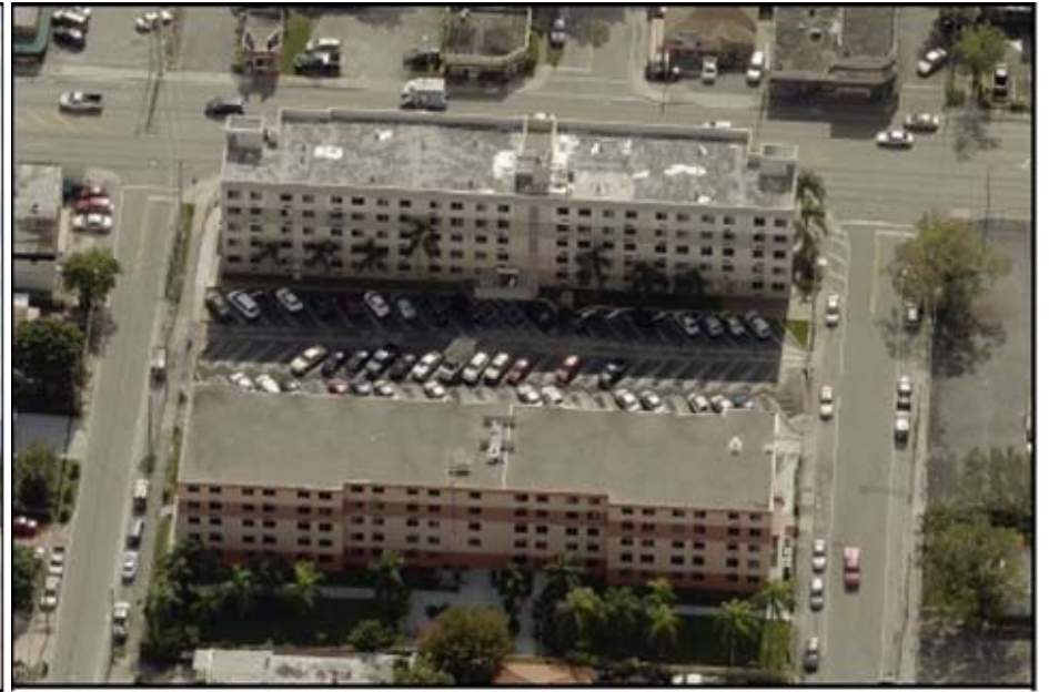
AERIAL VIEW OF SUBJECT PROPERTY (FACING SOUTH)
