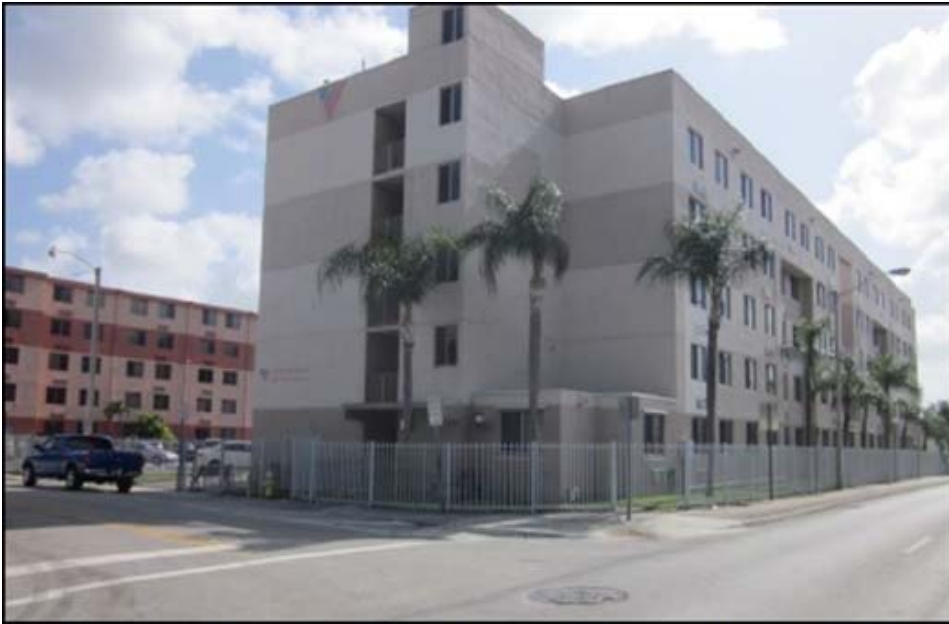
NORTHEAST VIEW OF SUBJECT BUILDINGS FROM N.W. 7TH STREET
